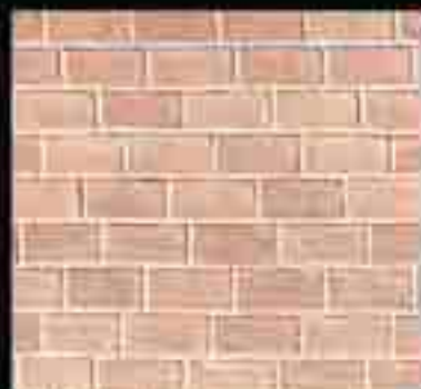
M-004 - Cordeau joint (Laidier joint)
