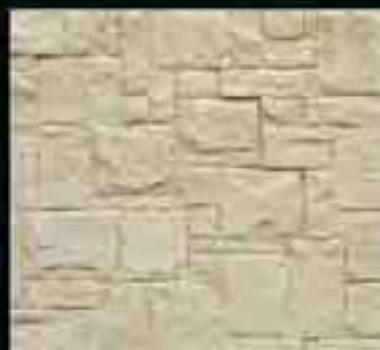
MA 117 - Close to camera / Thick stone base
